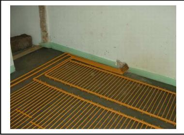
The principle of cooling the body instead of the entire air in the room means that the climatic wall/floor has much less energy consumption than normal air conditioners and therefore has a much lower running costs. In addition, the cooling energy can also be used for preheating your hot water. The climatic wall is very effective for use in attic apartments, loft extensions and buildings with flat roofs as it maintains the room climate even when the sun is burning down on the roof.
